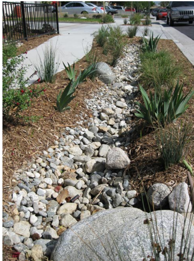
The street swale works as part of a system to capture and filter water before sending it down to the aquifer—away from the street.
